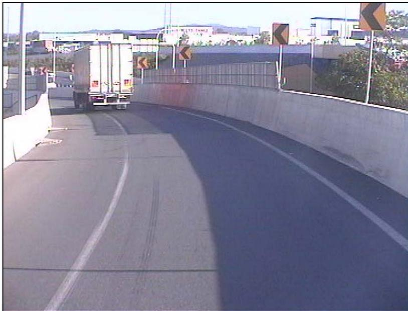
**FIGURE 2 Sight Distance Widening on Southbound Ramp between the Port of Brisbane Motorway and the Gateway Motorway**
