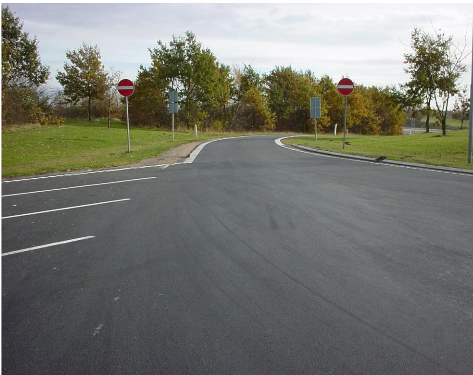
FIGURE 4: “Fish Trap Design Principle” that invites the driver to enter. But in this case it has been used wrongly because it is an exit that invites the driver to enter. Only enterings should be given this fish trap design while exits should be invisible or designed to give a “refuse” signal to the drivers
