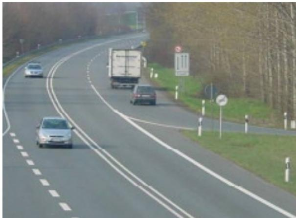
**Figure 3** Start of the two-lane passing section with lane addition at partially grade separated junction
