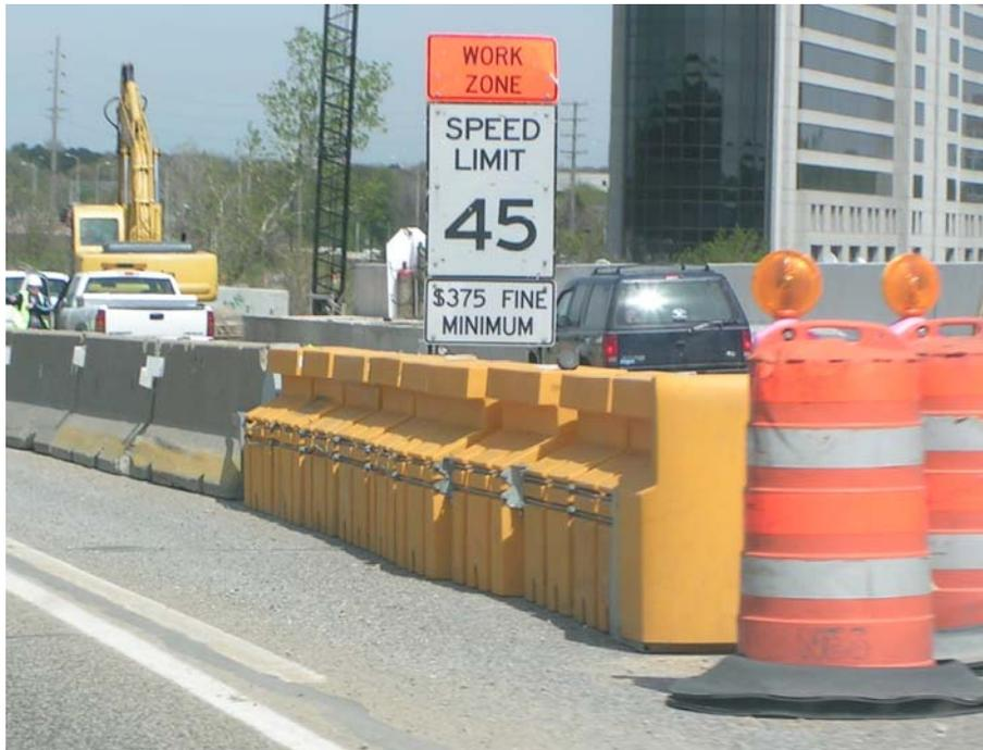
FIGURE 4 MOVEABLE CONCRETE BARRIER WITH ATTENUATOR
