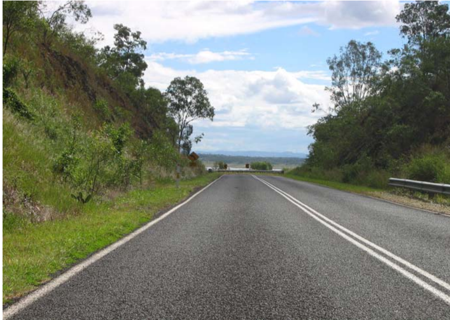
FIGURE 5 Wivenhoe–Somerset Rd: approach to R150 horizontal curve in southbound direction
