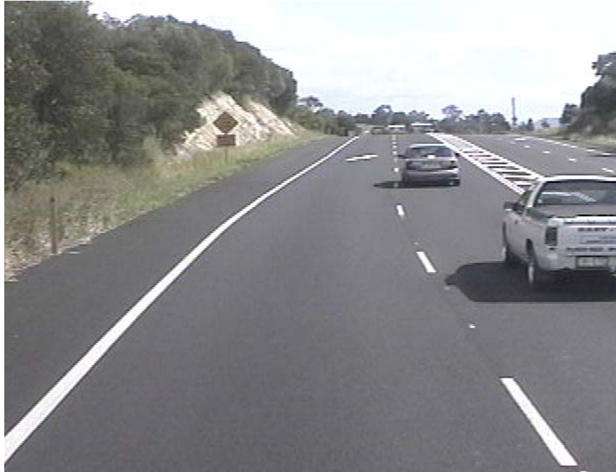
FIGURE 3 Bruce Highway at Federal: End of northbound overtaking lane
