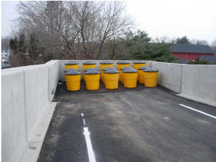
Photograph 5 – TER Terminus on Mechanically-Stabilized Earthwall (MSE)
