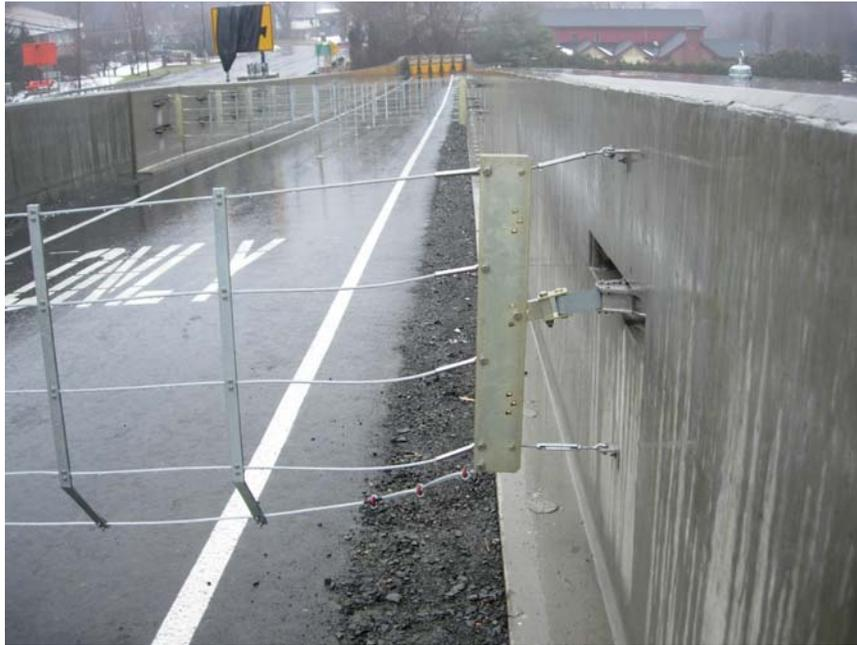
Photograph 4 – Crash Barrel Installation at TER Terminus.
