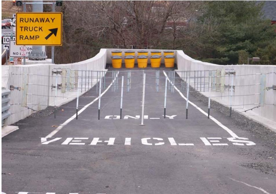
Photograph 2 – Installation of Stainless-Steel Arrestor Nets #2-#5
