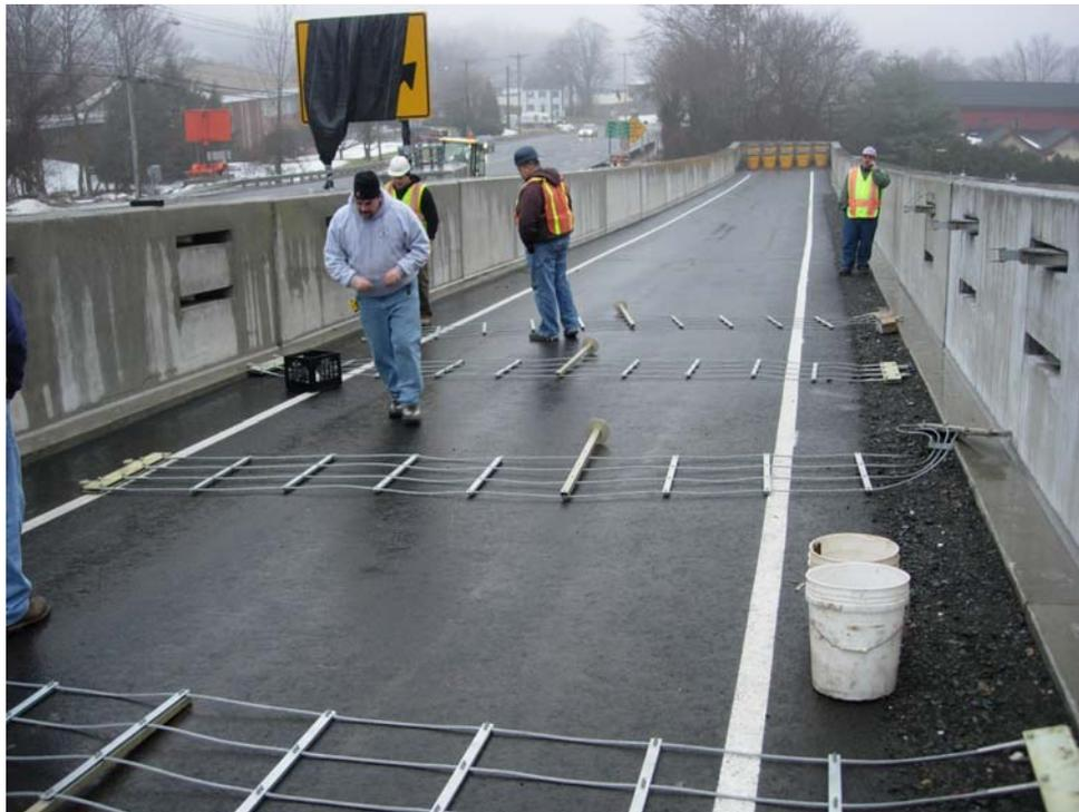
Photograph 3 – Arrestor Net #1 Connection to Mechanical Brake
