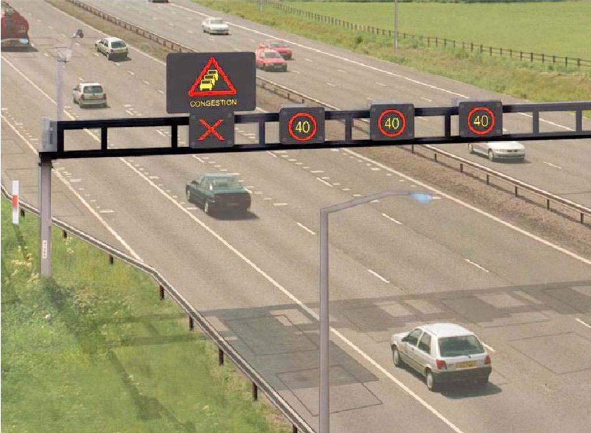
Figure 4 - Active Traffic Management as proposed for the M42 ATM project
