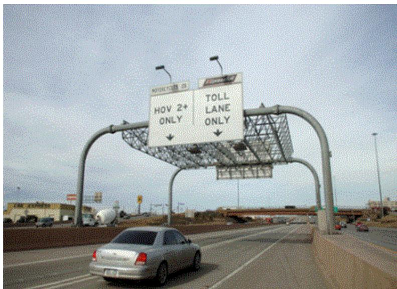
This photo shows an example of two types of managed lanes operating side by side: a high-occupancy vehicle (HOV) lane to the left and a toll lane to the right.
