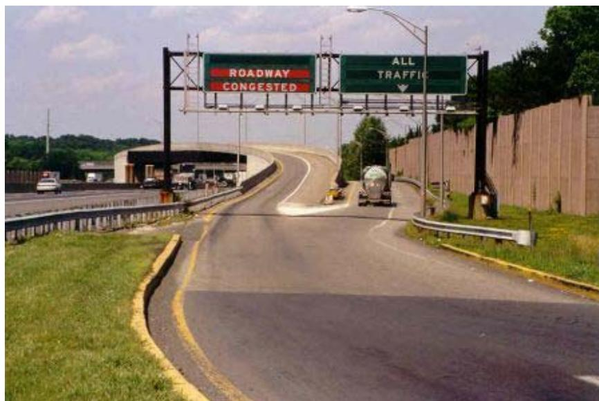
Dynamic message signs, such as this one on a U.S. interstate, are used on managed lanes to provide drivers with up-to-date traffic information.
